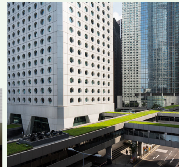
Green roofs on the footbridge at Central Portfolio.
